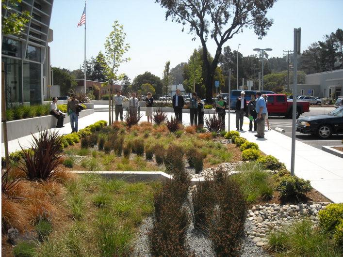
Figure 6-1. Bioretention Area. Source: City of Brisbane
