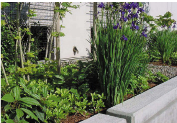
Figure 6-14: Close-up of Flow Through Planter. (Source: City of Portland)
