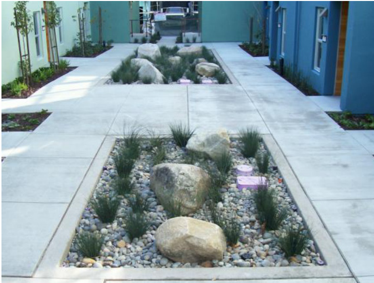
Figure 6-8: At-grade flow-through planter. Source: City of Emeryville
