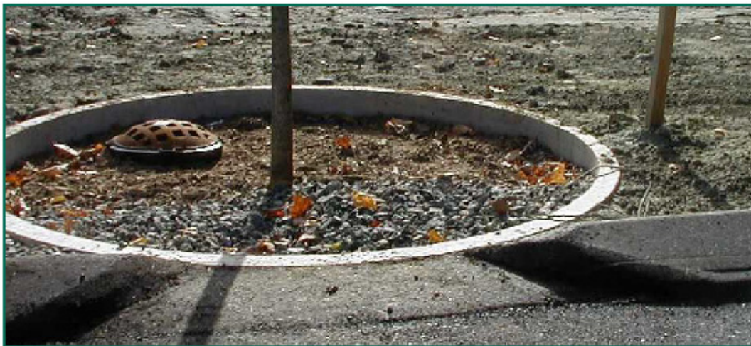
Figure 6-16: Non-proprietary Tree Filter with Overflow Bypass. Source: University of New Hampshire Environmental Research Group, 2006
