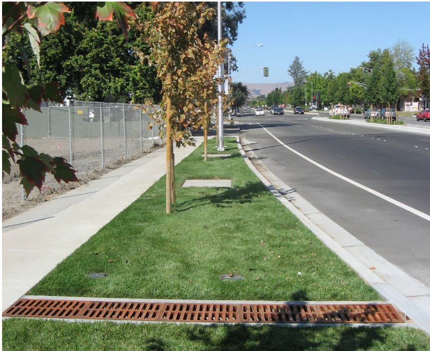
Figure 6-15: Non-proprietary tree well filters in Fremont use bio-retention soils with an infiltration rate of 5 to 10 inches per hour. Spacing the units closely together provides a total tree well filter surface area that is 4 percent of the impervious surface area from which stormwater runoff is treated.
