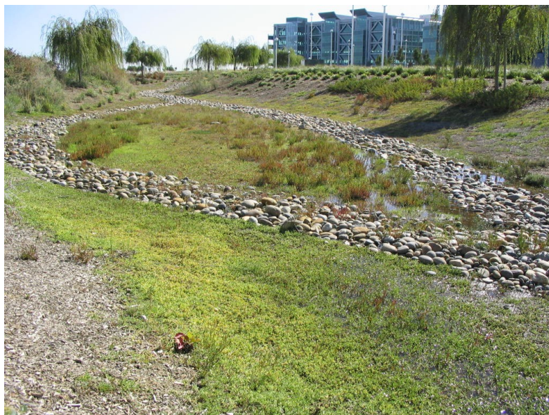
Figure 6-24: Extended Detention Basin. Photograph courtesy of Bill Southard (DES Architects and Engineers)
