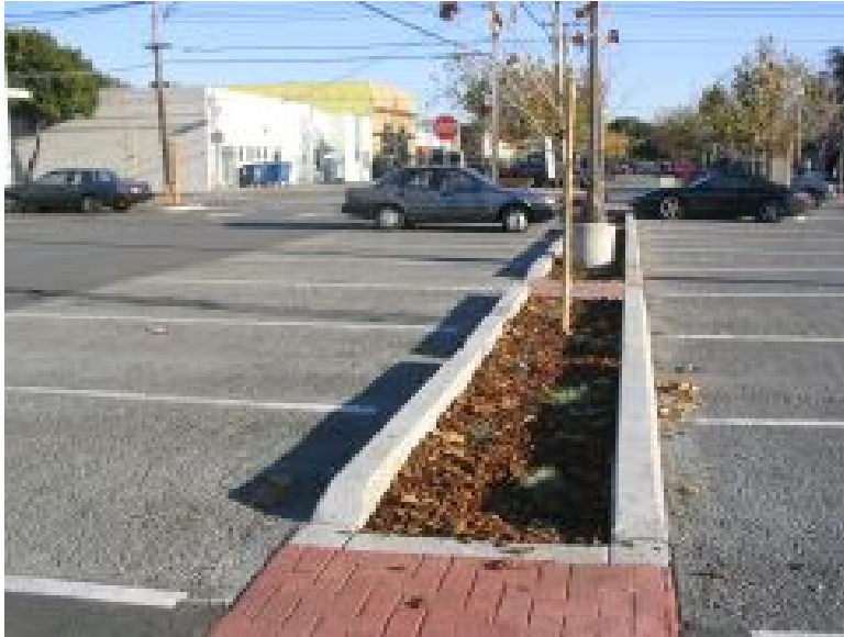
Figure 6-28: The City of Menlo Park used permeable concrete for parking stalls and standard paving in the drive aisles in this public parking lot.
