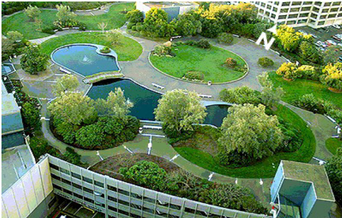
Figure 6-41: Intensive Green Roof, Kaiser Center Parking Garage, Oakland
