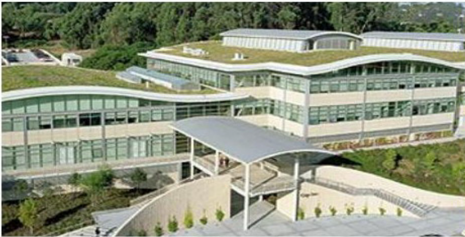
Figure 6-40: Extensive Green Roof at Gap Headquarters, San Bruno (William McDonough & Partners)
