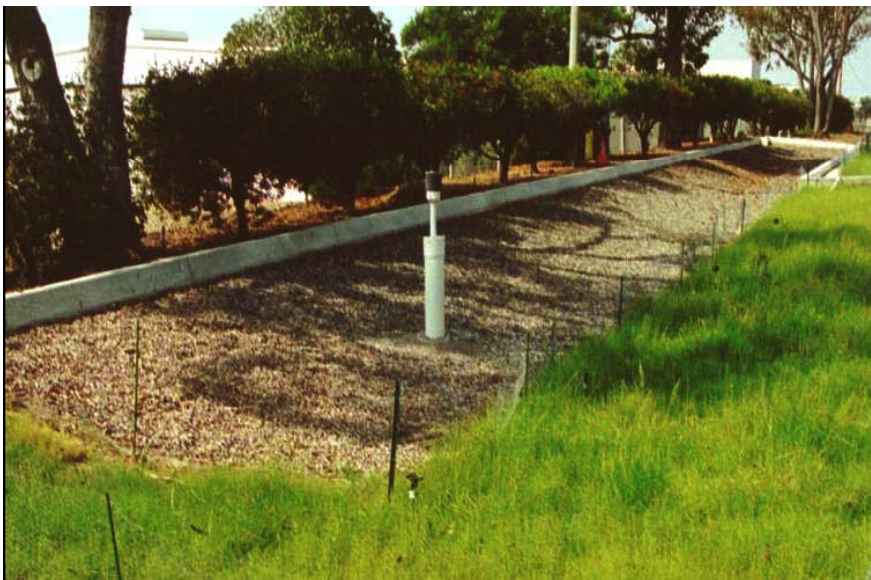
Figure 8-5: Infiltration Trench (Source: California Stormwater Quality Association)
