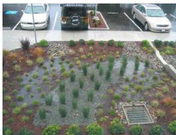
Rain garden collects and filters parking lot runoff in Brisbane.
