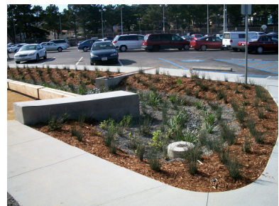
Bioretention area in Daly City.
