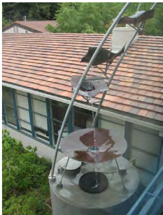
Figure 6-43: Rainwater is collected and used for flushing toilets at Mills College, Oakland.
