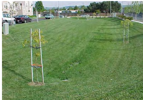
Figure 5-1: Extended Detention Basin, San Jose (example of a volume-based treatment measure)
