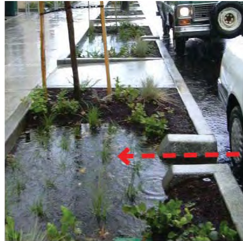
Figure 5-12: The side wings of this standard curb cut help retain the side slope grade on each side of the curb cut opening.
