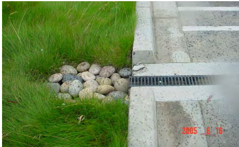
Figure 5-8: Cobbles are placed at the inlet to this stormwater treatment measure in Fremont, to help prevent erosion.
