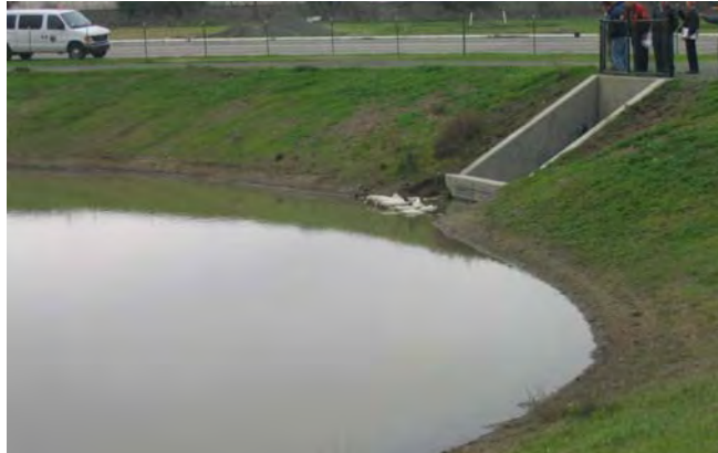
Figure 5-6: This detention pond provides both stormwater treatment and HM.
