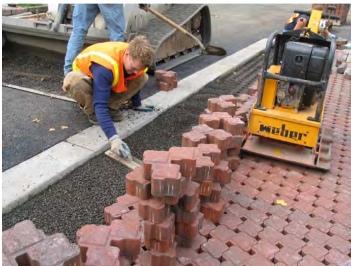
Figure 4-8: Installation of notched unit pavers in Portland, Oregon. Water infiltrates through notches between pavers. (Photo courtesy of City of Portland)
