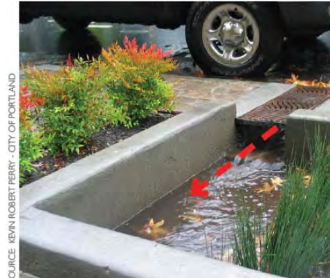
Figure 5-18: A grated curb cut allows stormwater to pass under a pedestrian egress zone to the stormwater facility.
