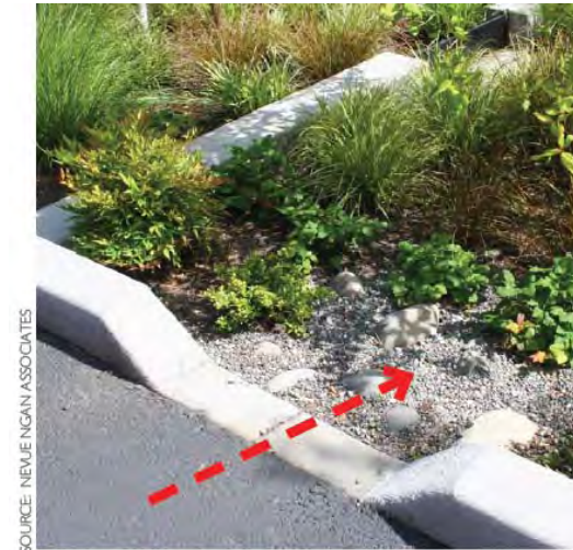
Figure 5-9: This standard curb cut at parking lot rain garden has 45 degree chamfered sides.
