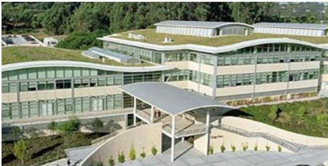
Figure 4-10: Extensive Green Roof at Gap Headquarters, San Bruno (William McDonough & Partners)
