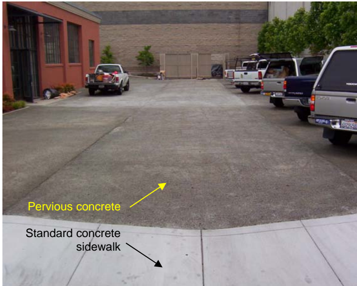
Figure 4-11: Pervious Concrete Parking Lot, Emeryville, California
