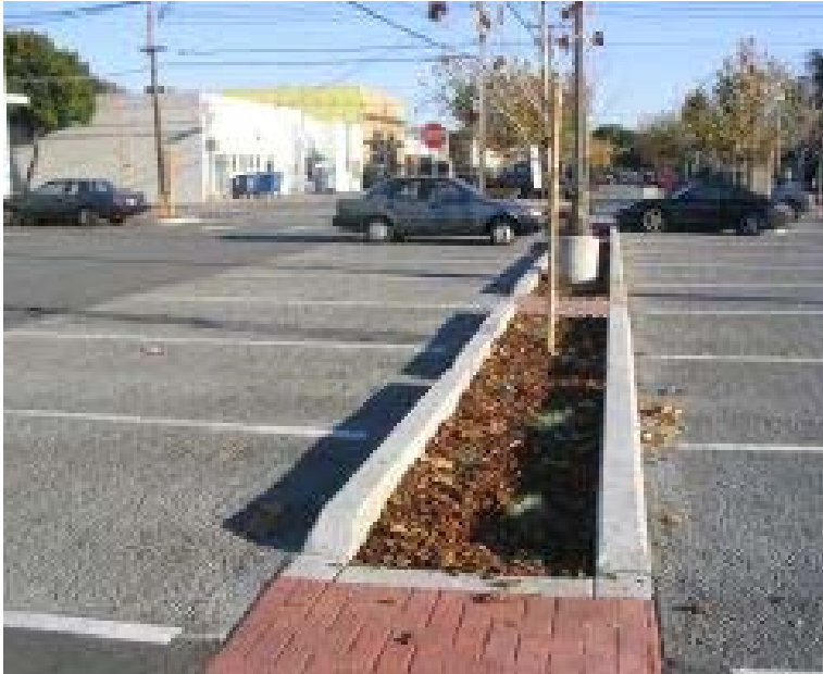
Figure 4-22: The City of Menlo Park used permeable concrete for parking stalls and standard paving in the drive aisles in this public parking lot.
