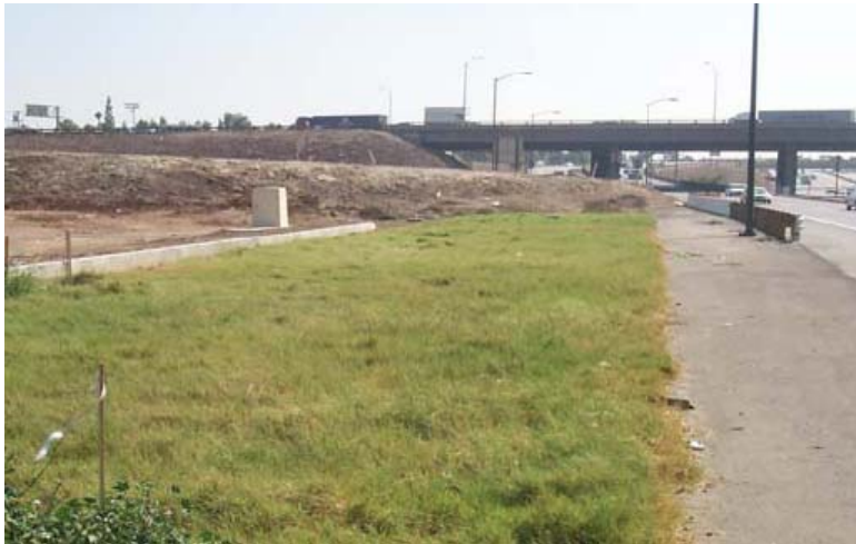
Figure 6-10: Roadside Vegetated Buffer Strip Source: www.cabmphandbooks.com
