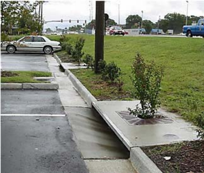
Figure 6-13: Tree Well Filter. Source: Americast, 2006. The use of this photo is for general information only and is not an endorsement of this or any other proprietary stormwater treatment device.
