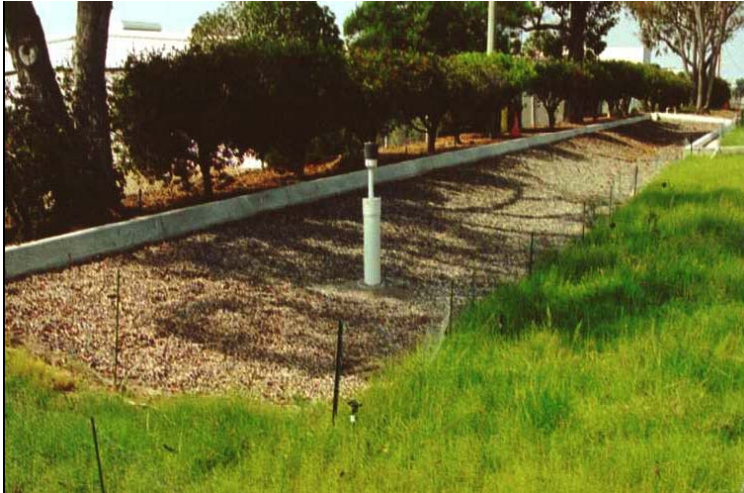
Figure 6-27. Infiltration Trench. Source: CASQA, 2003
