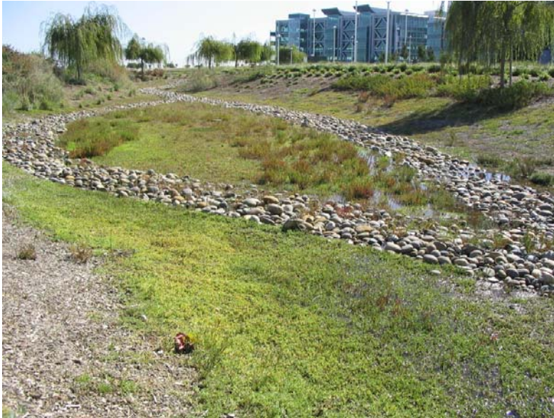
Figure 6-30: Extended Detention Basin. Photograph courtesy of Bill Southard (DES Architects and Engineers)
