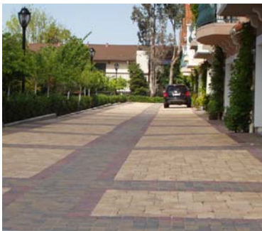
Ungrouted modular pavers promote infiltration, Redwood City
