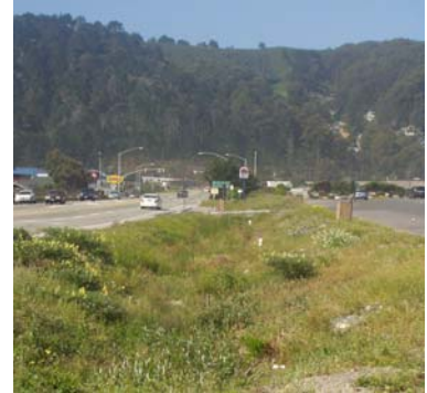
Roadway drains to vegetated swale, Pacifica
