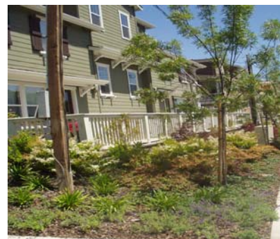
Figure 5-2: Vegetated Swale, City of San Mateo (example of a flow-based treatment measure)
