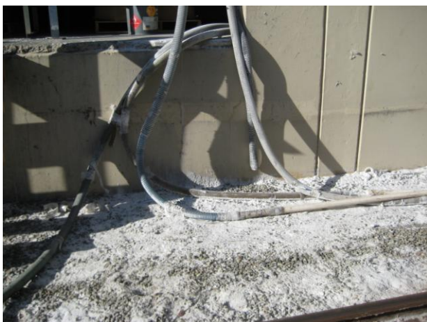
Photo 1a. Exterior of Metro Poly, 2009.
