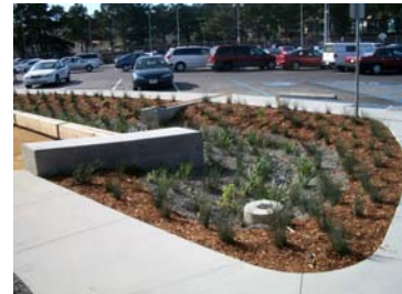
Bioretention area in Daly City collects and filters runoff from adjacent impervious surfaces.
