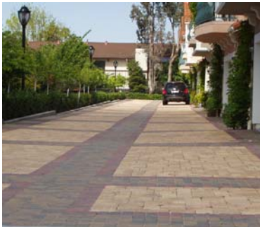
Ungrouted modular pavers promote infiltration, Redwood City
