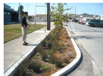
Vegetated swale collects and filters road runoff in San Bruno.
