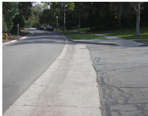
Figure 2-24: A concrete valley gutter allows water to flow through an intersection on the surface. The landscape system in the background is a good candidate for a vegetated swale retrofit.
