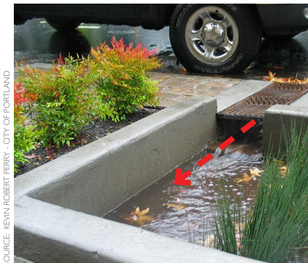
Figure 5-36: A graded curb cut allows stormwater to pass under a pedestrian egress zone to the stormwater facility.
