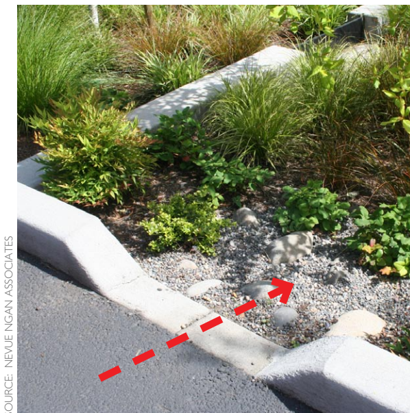
Figure 5-32: A standard curb cut allows stormwater runoff to enter a parking lot rain garden. This curb cut has 45 degree chamfered sides.
