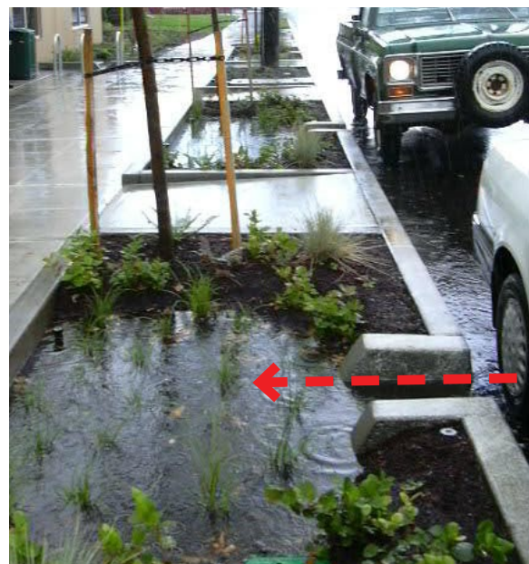
Figure 5-33: A standard curb with wings allows stormwater runoff to enter a stormwater facility. The wings help retain the side slope grade on each side of the curb cut opening.
