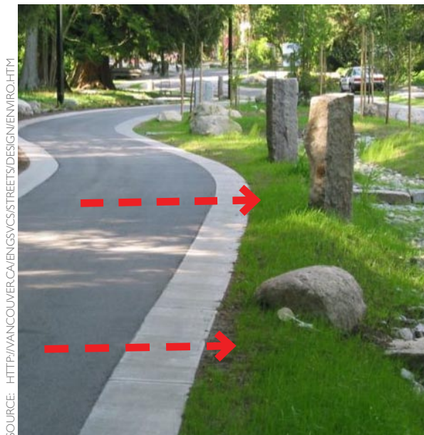
Figure 5-34: This flush concrete curb allows stormwater runoff to enter, evenly distributed, within a vegetated swale.
