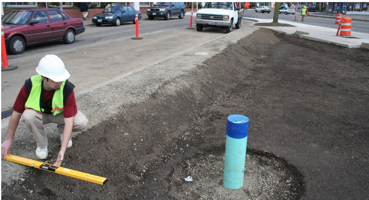
Figure 5-56: The design team should be on-site regularly during the grading process to determine whether or not the grading is consistent with the plans, and if necessary, work with the contractor to make field adjustments.
