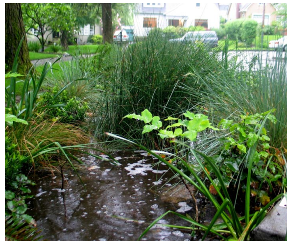
Figure 1-20: Landscape-based stormwater facilities, such as this stormwater curb extension, can capture urban debris before it gets into creeks and other waterways.
