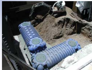
Cisterns installed underground
