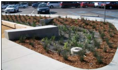
Bioretention system in Daly City
