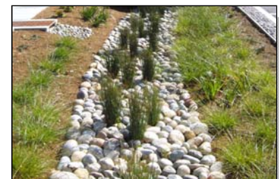
Bioretention system in Burlingame
