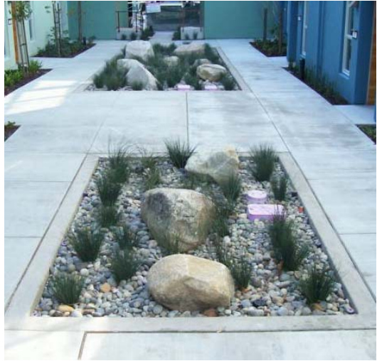
Figure 3-5: Flow-through planters in a dense, urban setting (Source: City of Emeryville)
