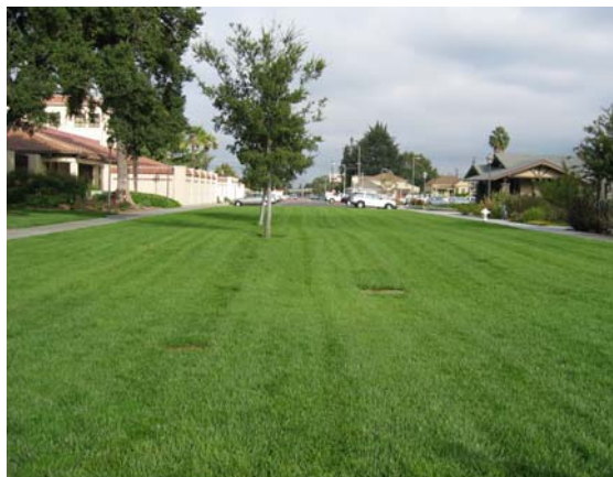
Figure 3-2: Turf block fire access road, Santa Clara University, Santa Clara
