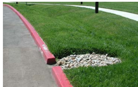
Figure 3-4: Cobbles help prevent erosion as stormwater enters treatment measure at Legacy Tech Park in San Jose. (Photo credit: RBF Consulting)
