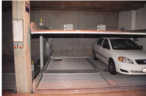
Figure 4-7: Parking Lifts in Parking Garage, Berkeley (photograph courtesy of City of Berkeley)
