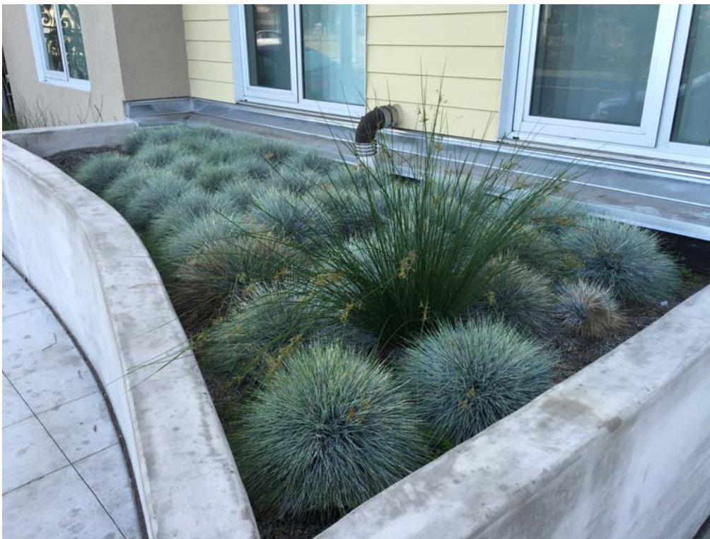
Figure 6-14: Close-up of Flow Through Planter with flow spreader. (Source: City of Emeryville)
