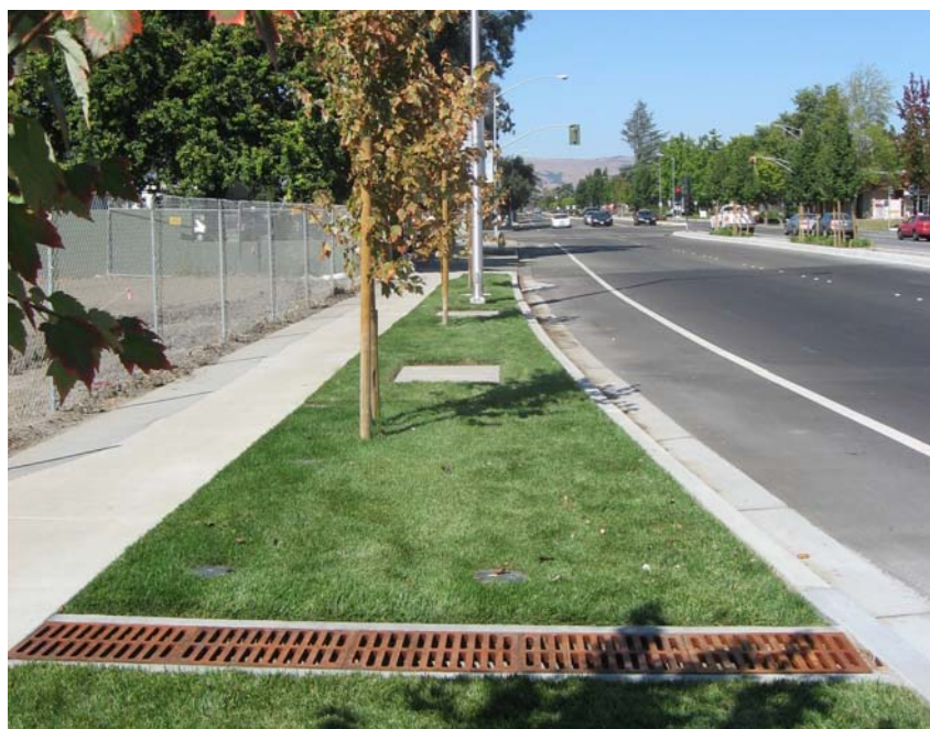
Figure 6-15: Non-proprietary tree well filters in Fremont use bio-retention soils with a long-term minimum permeability of 5 inches per hour. Spacing the units closely together provides a total tree well filter surface area that is 4 percent of the impervious surface area from which stormwater runoff is treated.
