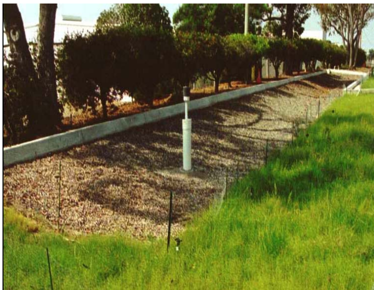
Figure 6-19. Infiltration Trench. Source: CASQA, 2003
