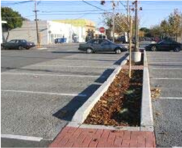
Figure 6-26: The City of Menlo Park used pervious concrete for parking stalls and standard paving in the drive aisles in this public parking lot.
