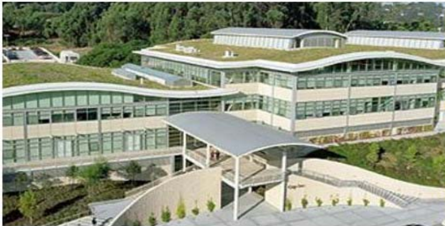
Figure 6-37: Extensive Green Roof at Gap Headquarters, San Bruno (William McDonough & Partners)
