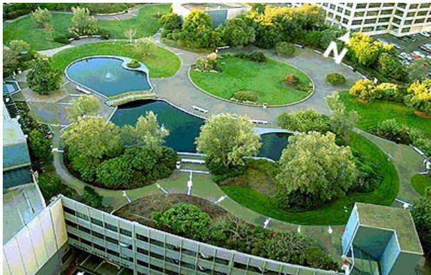
Figure 6-38: Intensive Green Roof, Kaiser Center Parking Garage, Oakland
