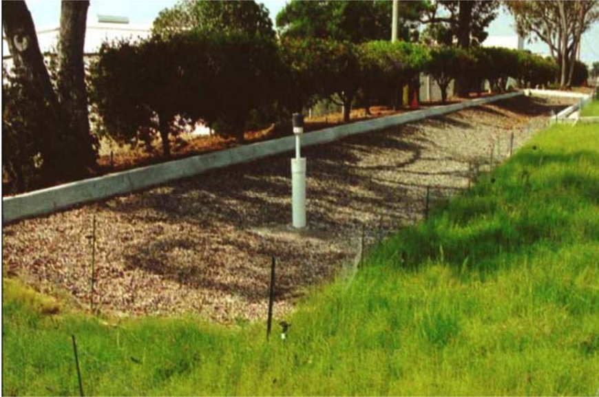
Figure 8-4: Infiltration Trench (Source: California Stormwater Quality Association)
