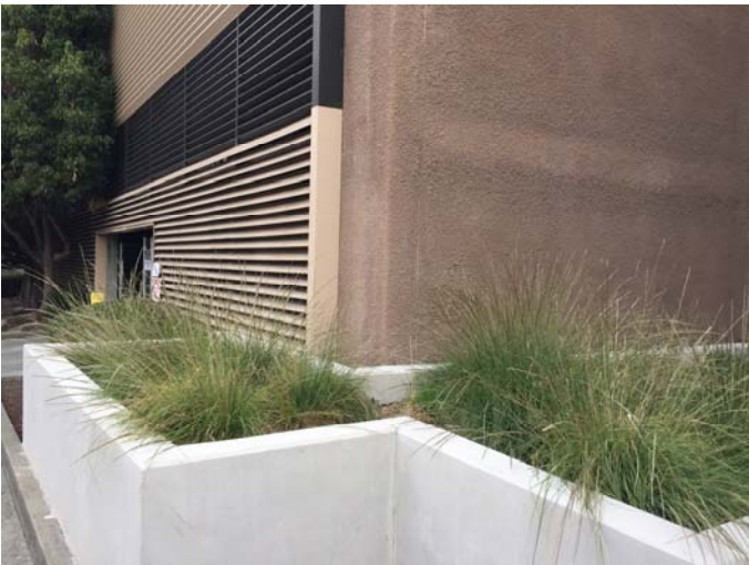
Figure 8-2: Flow through planter in Emeryville
