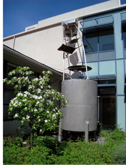
Figure 8-7: Rainwater Harvesting Cistern in Oakland at Mills College
