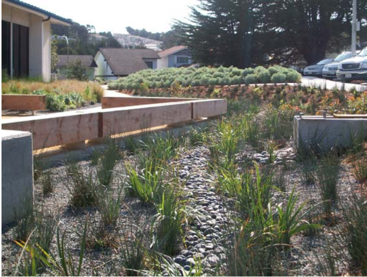
Figure 8-1: Bioretention Area in Daly City
