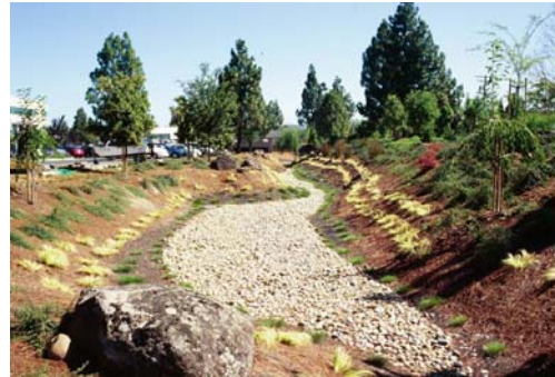
Figure 8-5: Extended Detention Basin, Palo Alto
