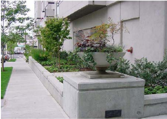
Flow-through planters are designed to treat and temporarily detain runoff without allowing seepage into the underlying soil. They typically receive runoff via downspouts leading from the roofs of adjacent buildings.
