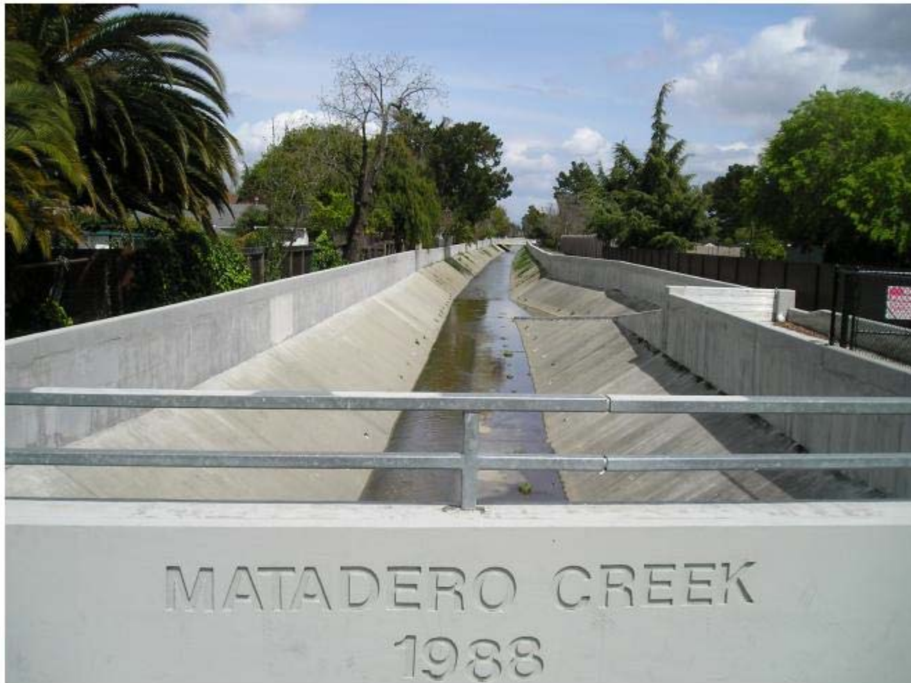
Concrete Lining with Floodwall – Matadero Creek
