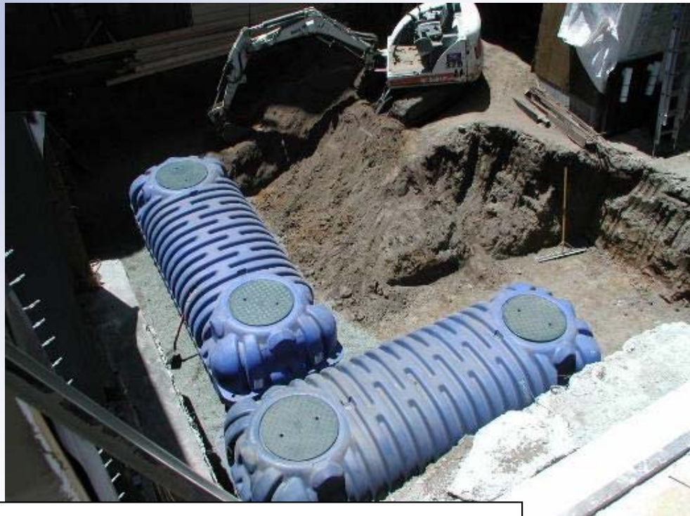
Cisterns installed underground
