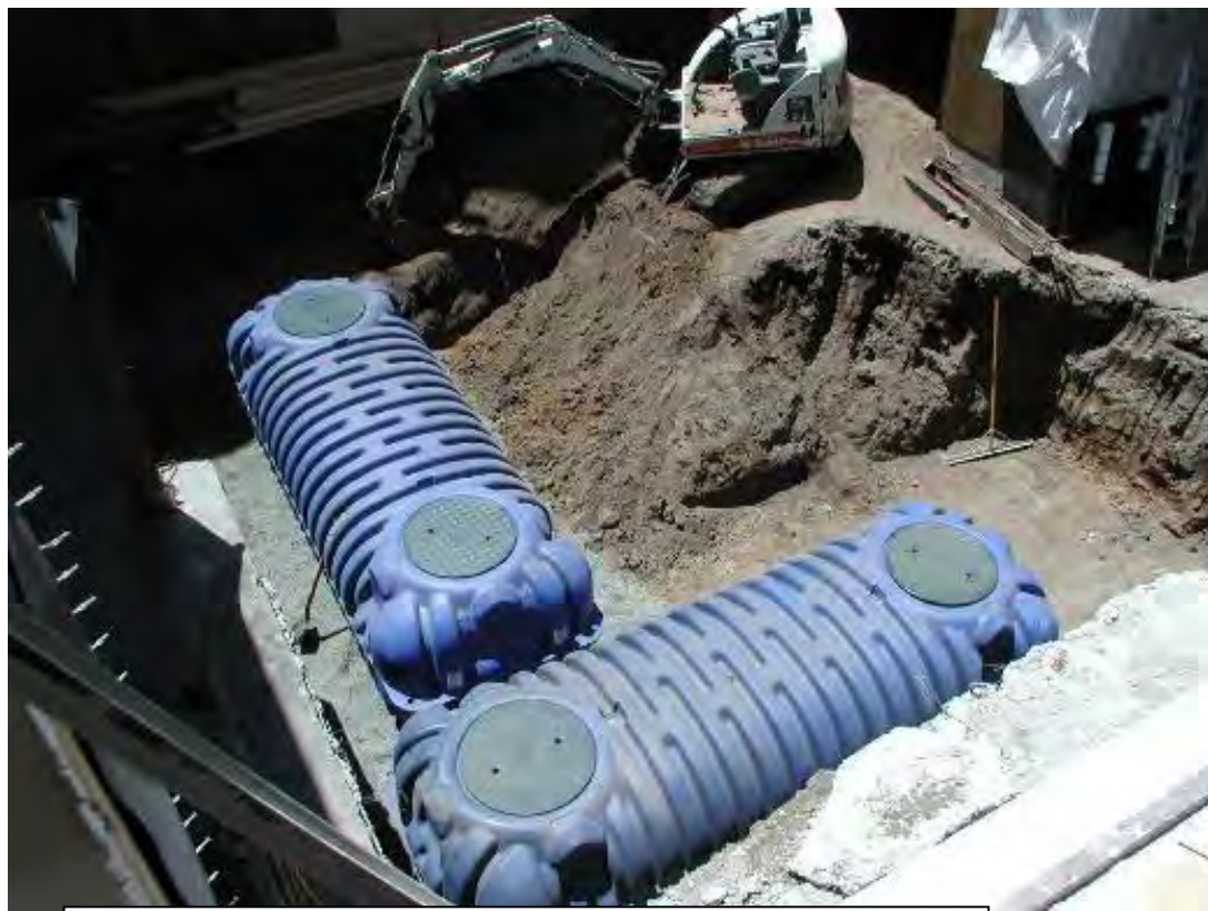
Cisterns installed underground
