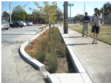
A vegetated swale in San Bruno slows and treats runoff from roadway.
