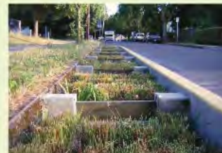
▲ EXAMPLE: This neighborhood connector incorporates a bio-retention planter with check dams to reduce velocities on a sloping street.
