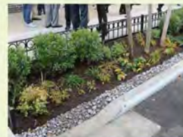
▲ The gravel band along the curb helps to dissipate stormwater runoff flows into the planter.
