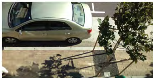
▲ Stormwater trees can be linked together with pervious pavement, modular suspended pavement, and other techniques to expand runoff storage capacity.
