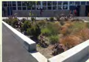
▲ This rain garden is graded very shallow to allow ponding of water, but it is not excessively deep or have steep side slopes. Ultimately this rain garden will perform better over time and will be easier to maintain.
