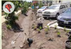
▲ This newly installed green infrastructure facility will have consistent problems with erosion control and plant health issues because of steep side slope conditions (steeper than 3:1 slope).
