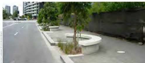
▲ These stormwater trees are flanked by seating areas. A metal capped inlet should be provided across the face of the planter to prevent vehicles from entering the planters.
