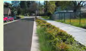
▲ A shallow green gutter is retrofitted along a rural residential street. The project also incorporated a pervious concrete sidewalk that now allows children to safely walk to a nearby elementary school.
