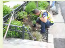
▲ As with other green infrastructure measures, stormwater tree planters will need to be maintained to remove debris and sediment and replant vegetation that declines.
