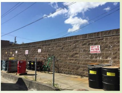
The fourth side has a 6 inch berm running the length of the containment area with a <u>4 foot</u> break at one end adjacent to a ramp for forklift access.
