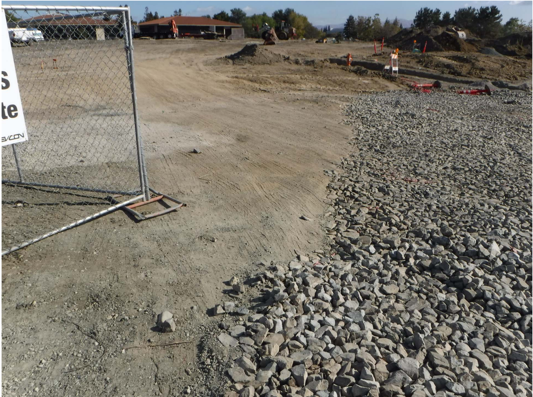
Site #2: Construction exit at large site during first inspection.
