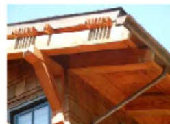
Building with copper flashing, gutter and drainpipe.
