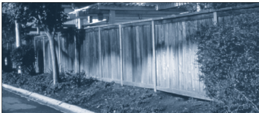
Damage to fencing from sprinkler irrigation.
