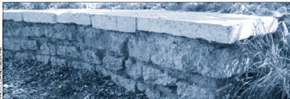
Reused concrete makes attractive benches, retaining walls, and raised planting beds.
