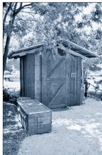
Garden shed made with salvaged lumber from deconstructed warehouses at Oakland Army Base.
