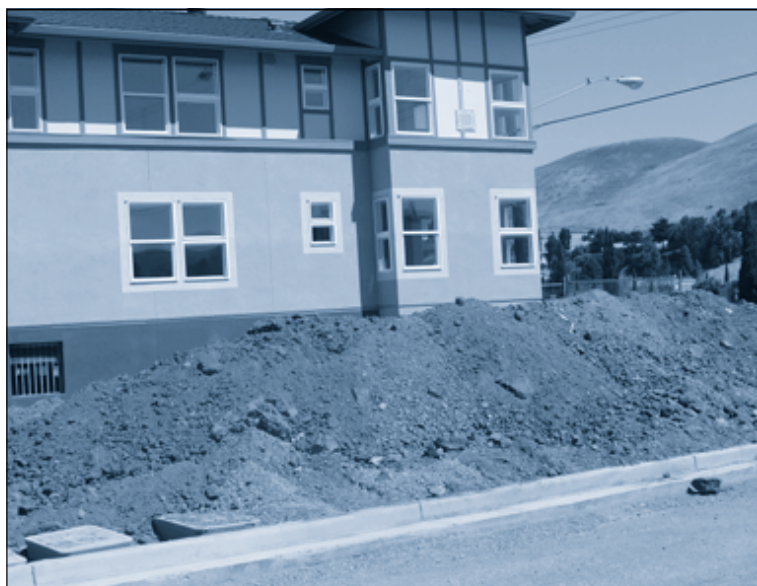
Topsoil has been removed and stockpiled before building construction for later re-use in the landscape.
