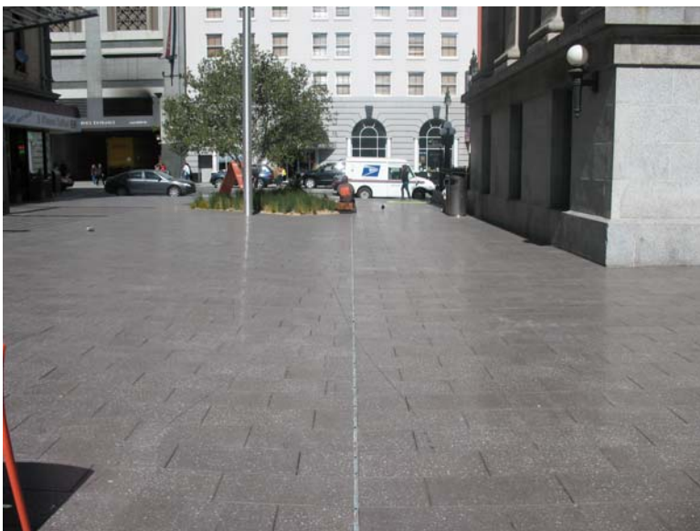
Mint Plaza: 1/2-inch slot drain (center); bioretention area (far end of plaza)
