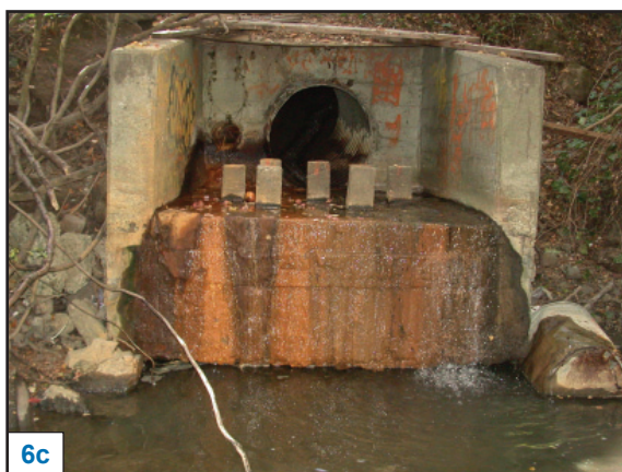
Figure 6. Illegal connections and illicit discharges: a) horse paddock encroaching on riparian corridor; b) pool backwash pipe entering creek; c) outfall with stains and residues; d) incision caused by historic burst water pipe.
