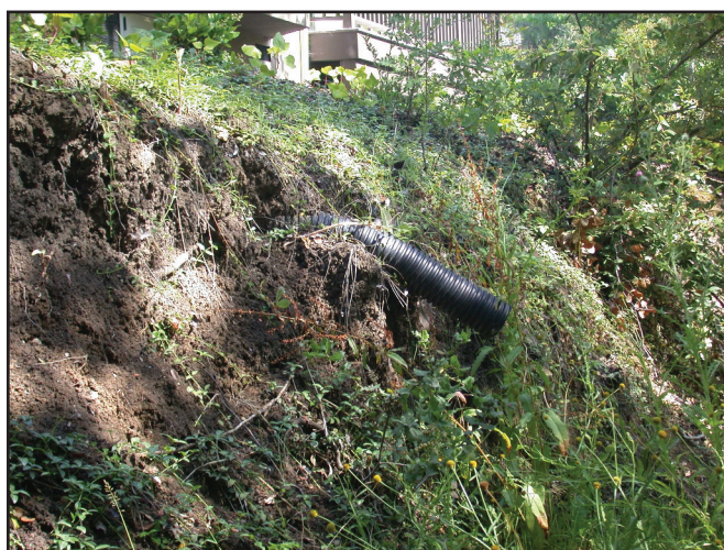
Figure 15. Streambank erosion caused by inappropriate landscape pipe placement and plantings.
