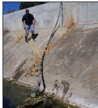
Figure 7. Water diversion pipe and pump.
