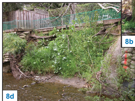
Figure 8. Infrastructure requiring repair: 8a) Hanging outfall; 8b) Outfall threatened by erosion; 8c) Erosion and aggradation burying an outfall; 8d) Failed saccrete threatens private property; 8e) Erosion threatens private property.
