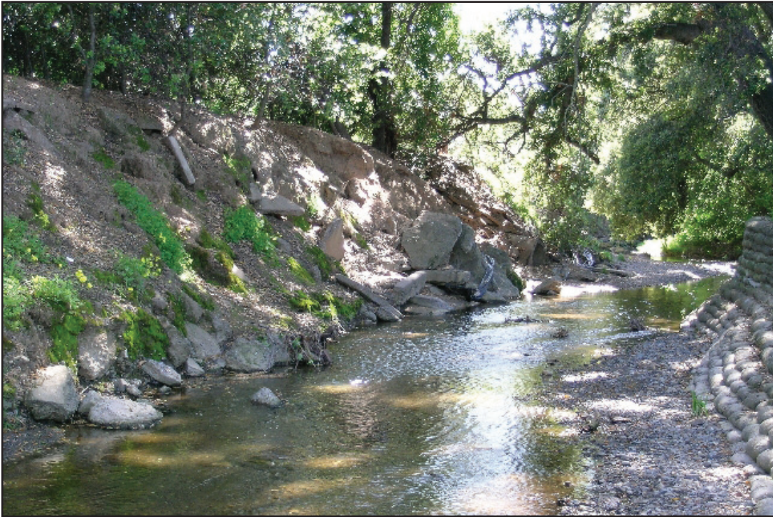
Figure 12. Failing streambank revetment and subsequent erosion.
