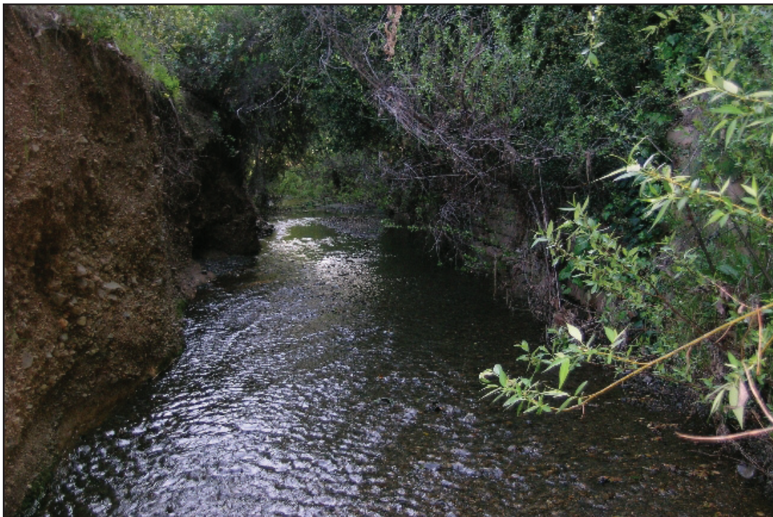
Figure 13. Bank scour resulting from hydromodification and channel engineering - the channel appears to have been straightened, and hardened on the opposite bank, thereby restricting flow and increasing its velocity, resulting in scour of the opposite bank.
