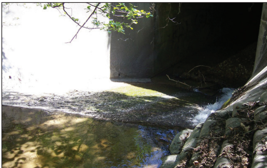
Figure 18. Highway culvert potentially acting as a barrier to fish passage.
