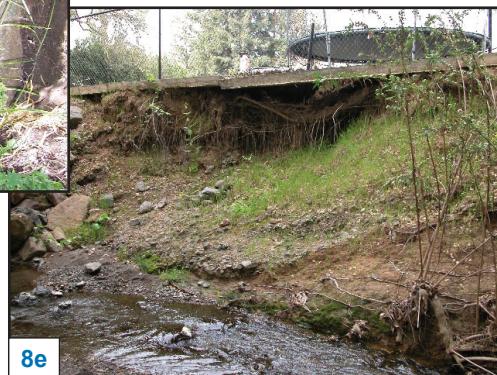
Figure 8. Infrastructure requiring repair: 8a) Hanging outfall; 8b) Outfall threatened by erosion; 8c) Erosion and aggradation burying an outfall; 8d) Failed saccrete threatens private property; 8e) Erosion threatens private property.
