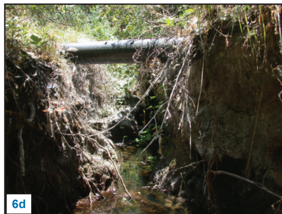
Figure 6. Illegal connections and illicit discharges: a) horse paddock encroaching on riparian corridor; b) pool backwash pipe entering creek; c) outfall with stains and residues; d) incision caused by historic burst water pipe.
