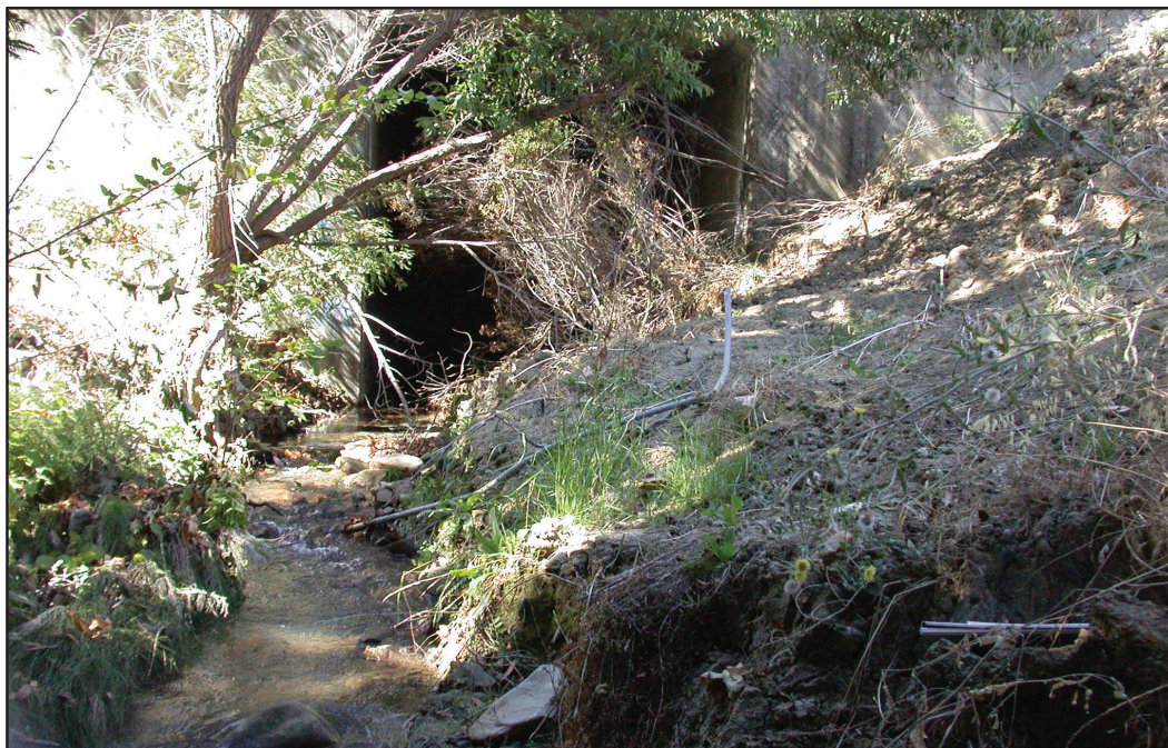
Figure 10. Landslide debris entering creek below a vineyard, blocking a large part of a road culvert and introducing high volumes of sediment to the stream.
