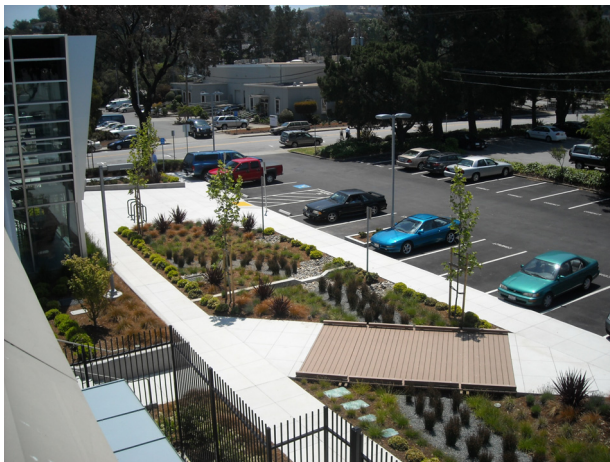
Rain garden/bioretention area at Brisbane City Hall's completed green parking lot
