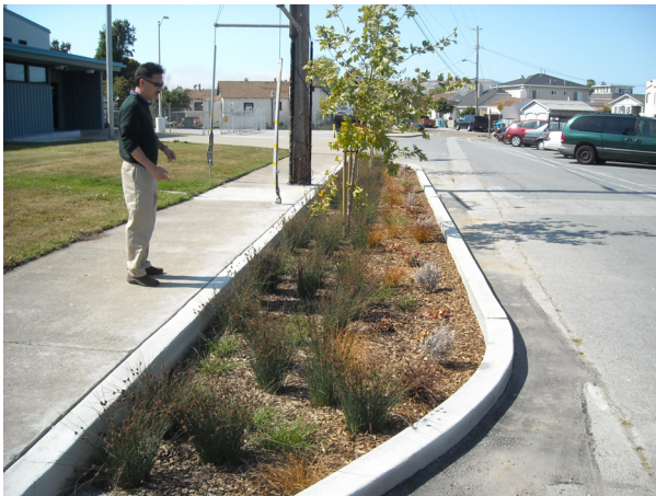
Stormwater curb extension, San Bruno's Belle Air/Third Avenue completed green street project
