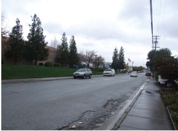
Figure 3-1. Bransten Road in San Carlos is the location of a potential pilot green street project.
