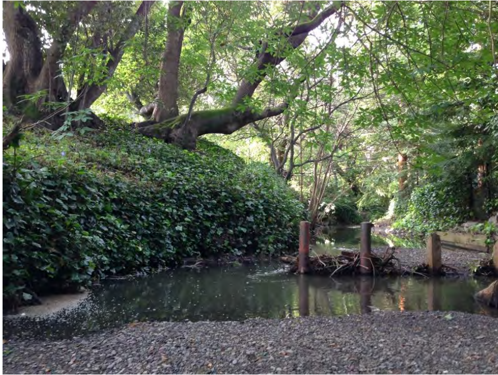
Figure 3. Downstream end of De Anza Park showing a large debris trapping structure.
