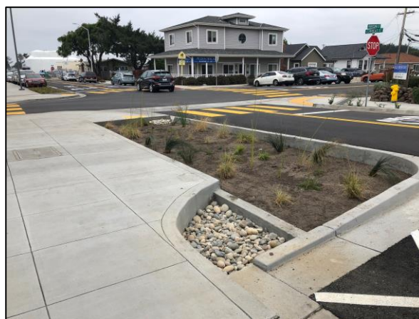
Figure 3-1. Completed Half Moon Bay Pilot
