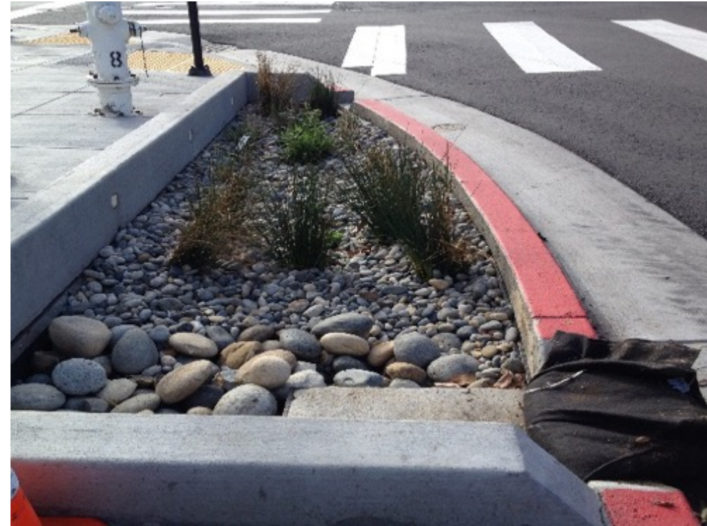
Rock and cobble mulch with temporary blockage of inlet during plant establishment in San Francisco
